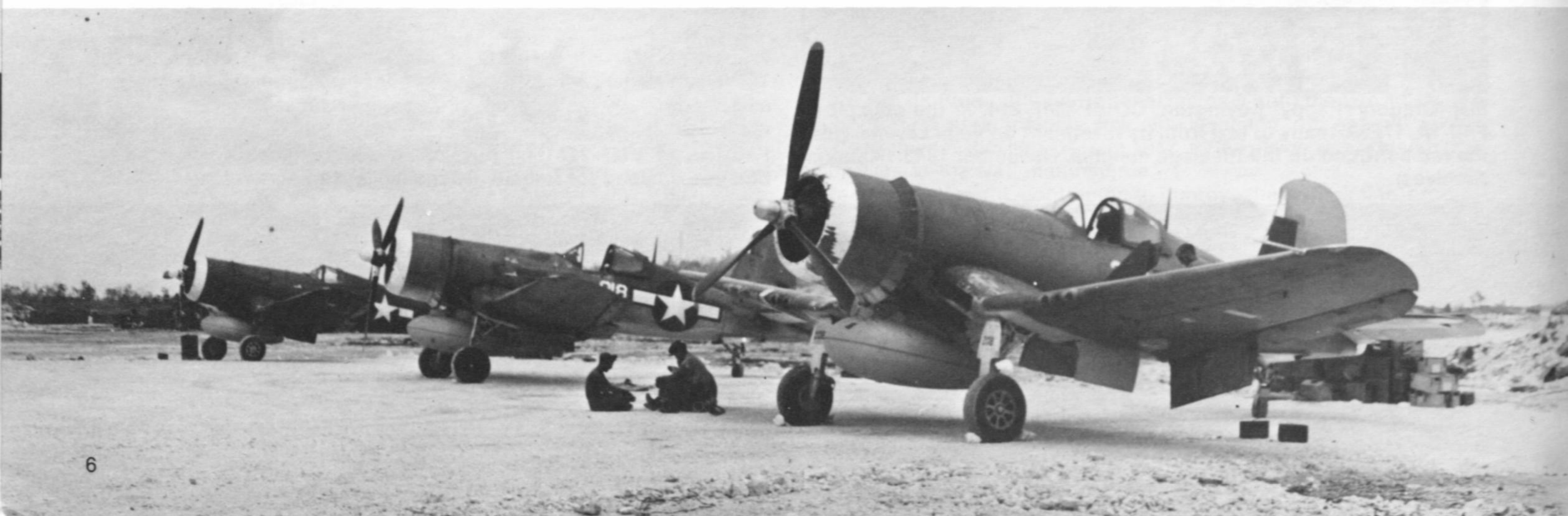
(Below) A white-nosed FG-1A, 14220, from VMF-114 is loaded with napalm (in the early-style drop tanks) for strikes against Japanese dug in on Bloody Nose Ridge on Peleliu, October 1944. (USMC)
